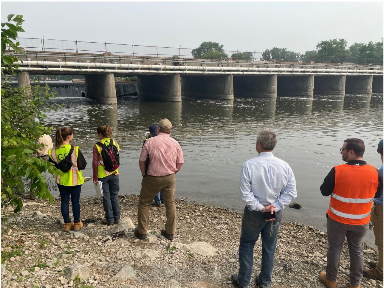
Figure 1: Project team meets on site at Flatrock Dam to discuss next phase of removal feasibility study. This study includes federal, state, and local partners who are advising a multidisciplinary team. Field study is beginning this summer and will be ongoing throughout 2023 and 2024.
