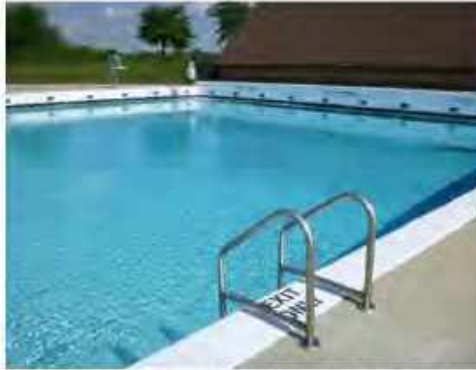
Image 17: Gutter Operating at Surge Weir Elevation
