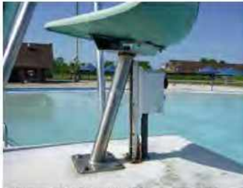
Image 30: Wave Pool Emergency Stop
