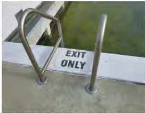
Image 22: Deep End Ladder Rails
