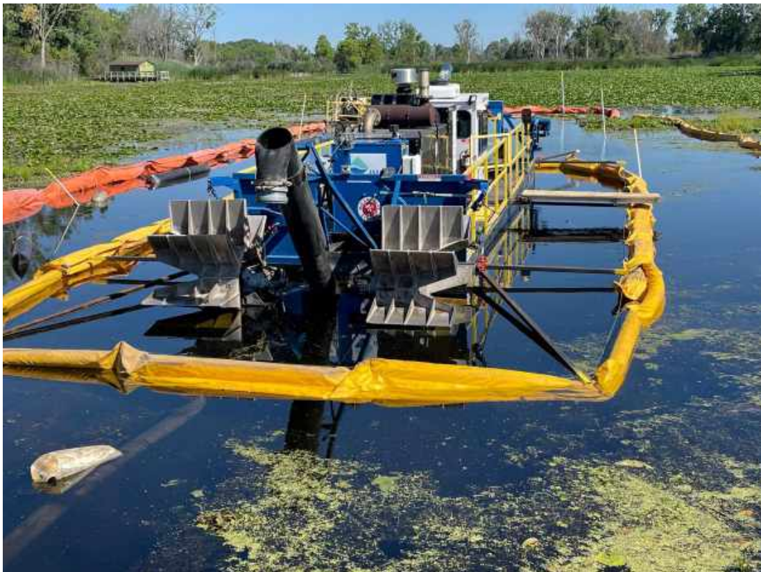
Figure 2: Marsh restoration dredge equipment working at Lake Erie Metropark.
