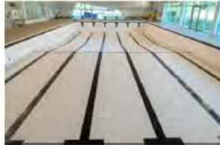
Myrtha Skin: Stainless Steel Rolls & Installation
