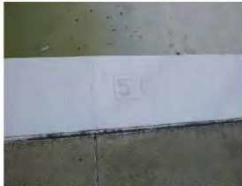
Image 27: Faded Depth Marking
