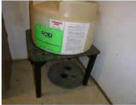
Image 69: Muriatic Acid Storage Tank & Stand
