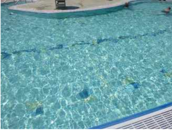
Expansion joint in pool area
