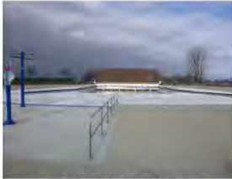
Image 24: Splash Pad Railing
