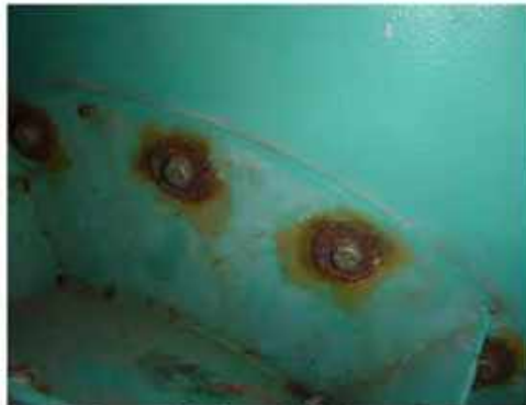
Image 85: Corroded Fasteners
