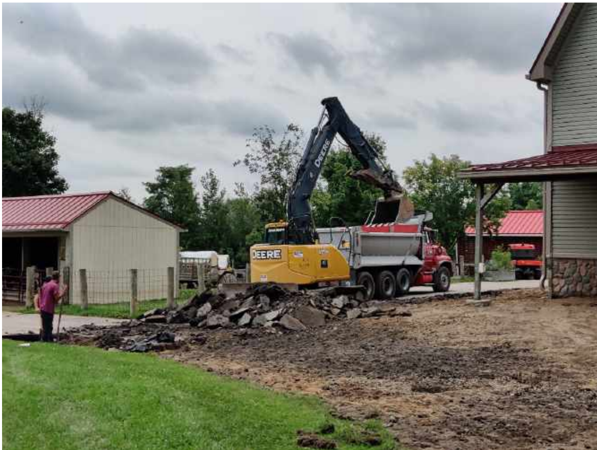
Kensington Farm Center – pathway paving project
