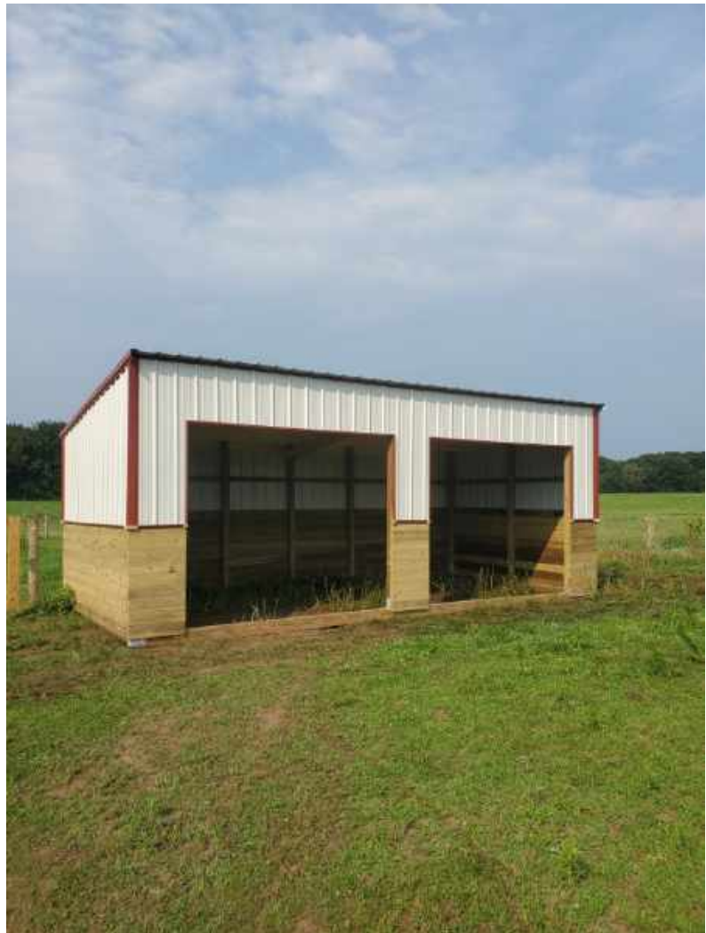
Wolcott Mill Metropark Farm Center New Horse Run-in Shed
