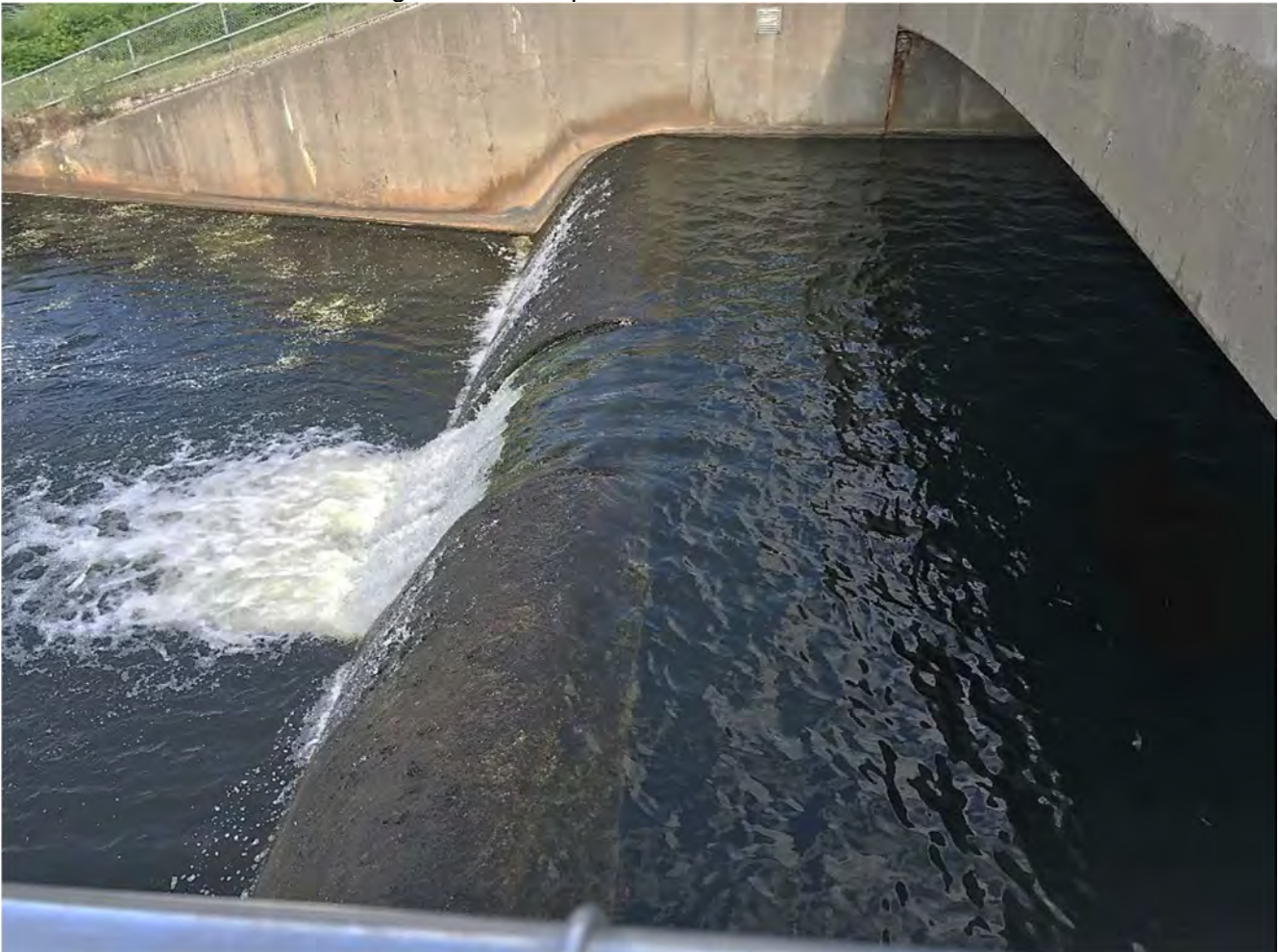
Upper Stony Lake Dam
