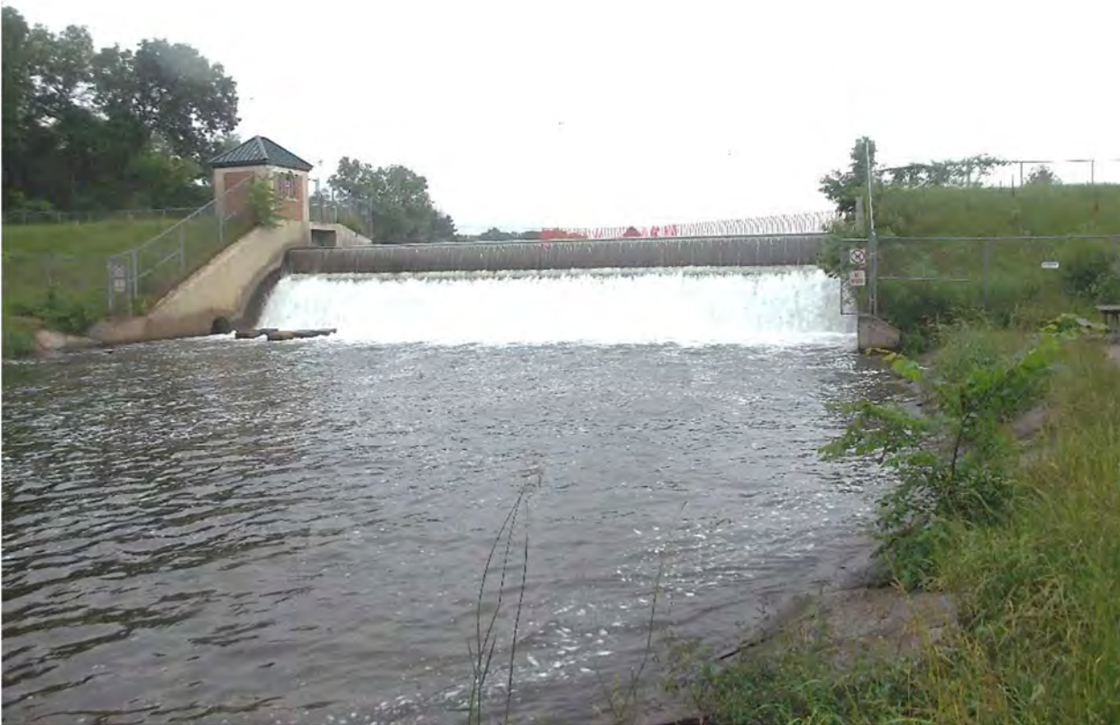
Kent Lake Dam
