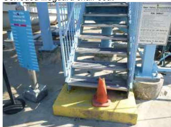
Slide entrance and caution cone
