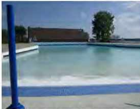
Image 86: Water Shy of Beach Entry Gutter
