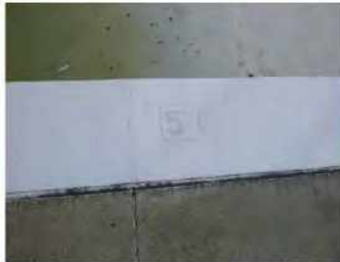
Image 27: Faded Depth Marking
