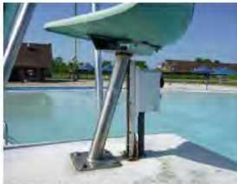
Image 30: Wave Pool Emergency Stop
