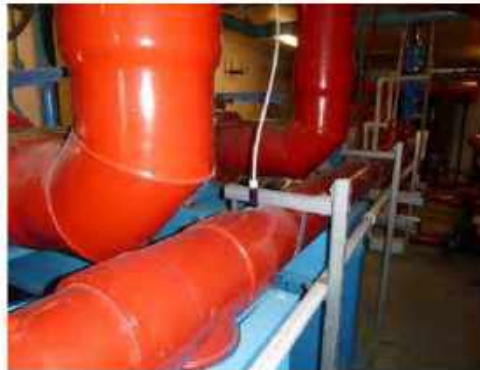
Image 72: Chemical Injection Tap
