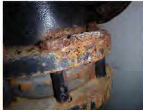
Image 38: Valve Corrosion
