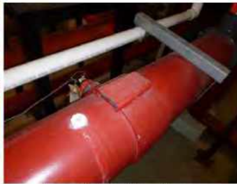
Image 48: Flow Meter Sensor
