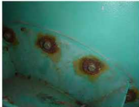
Image 85: Corroded Fasteners
