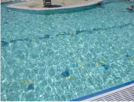
Expansion joint in pool area
