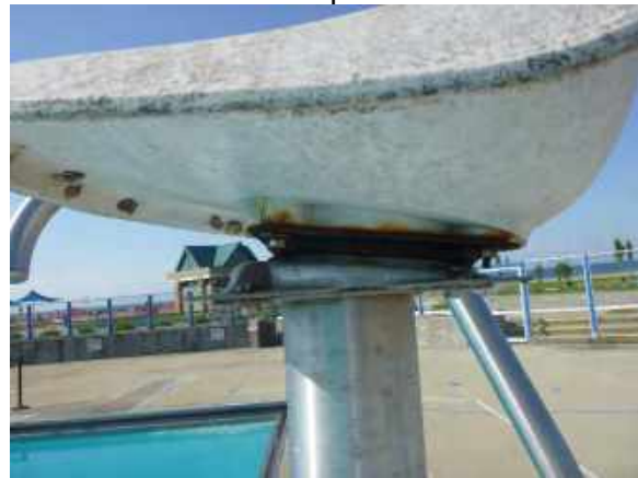
Corroded lifeguard chair seat
