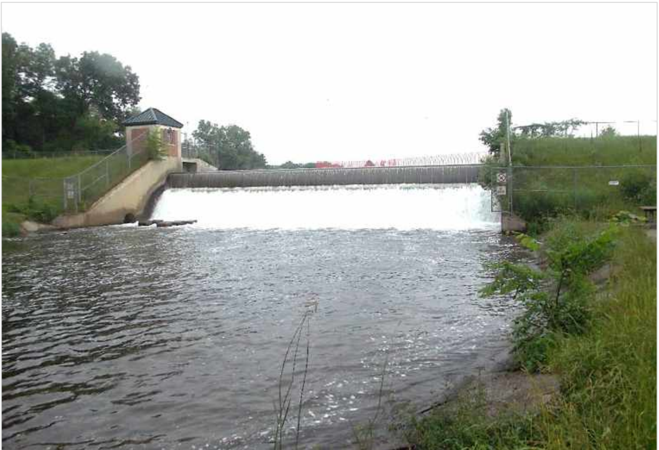
Kent Lake Dam
