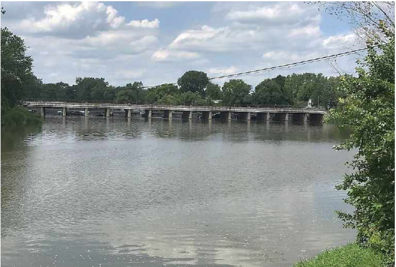
Flat Rock Dam
