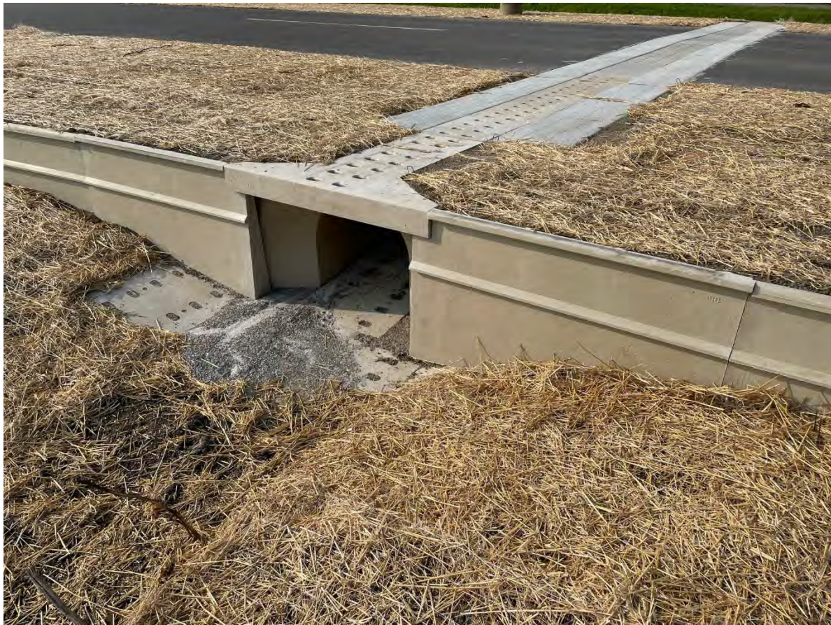
Figure 1: A wildlife crossing tunnel was recently installed on the entrance road at Lake St. Clair Metropark. This important project provides a pathway for reptiles and amphibians, especially slow-moving turtles, and a safe passage across the lane as they move between the Point Rosa and Black Creek marshes. This project will serve as a pilot and help Natural Resources staff determine the efficacy of this installation and provide guidance for future similar projects.
