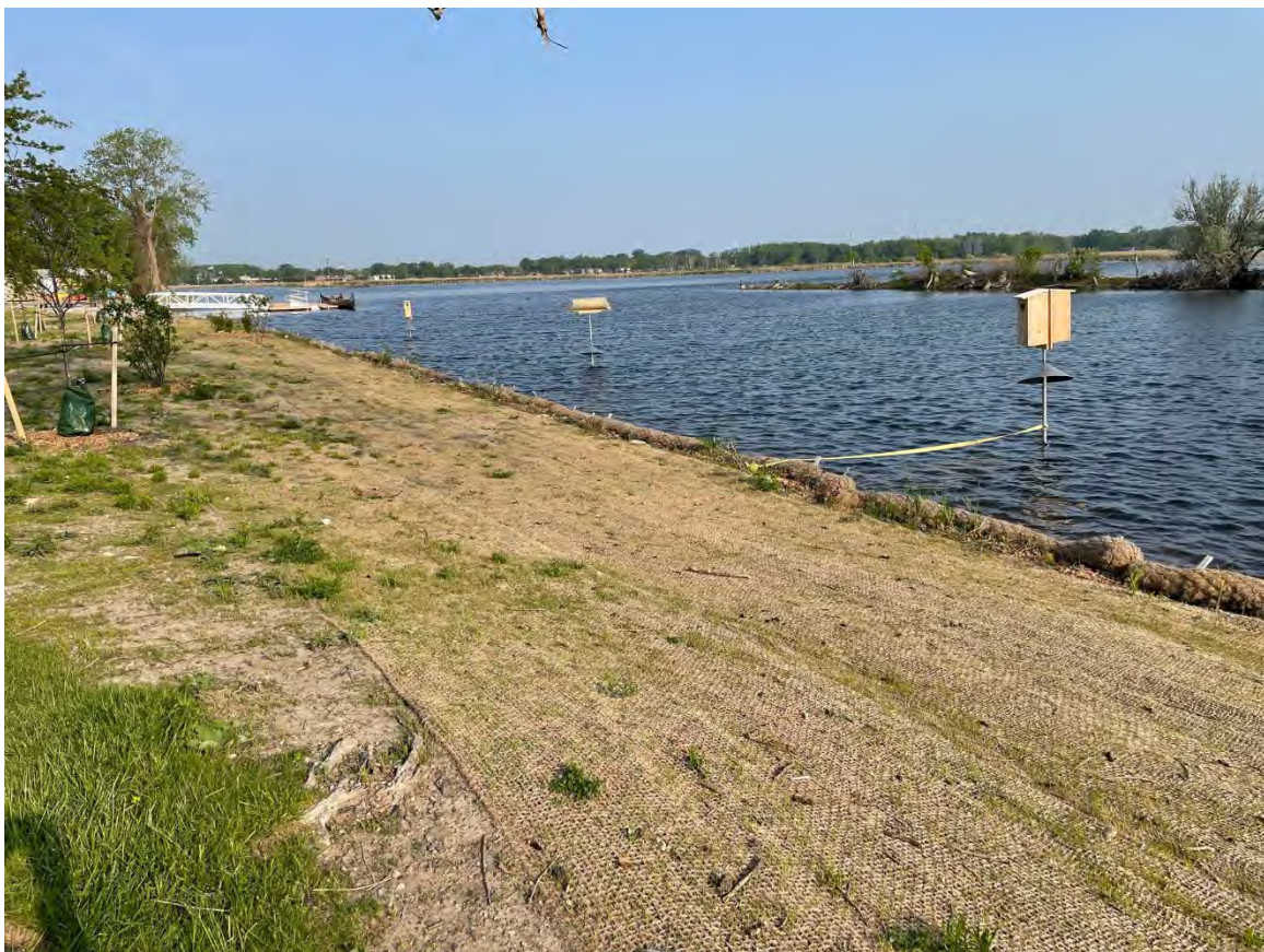
Figure 4: The Natural Shoreline project at Lake St. Clair Metropark, on the Black Creek Marsh, is nearly complete. Trees and shrubs have been planted, and seeded areas are beginning to sprout and grow. 105/219
