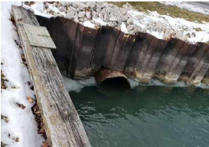
Exhibit 1. Example of Submerged Outfall
