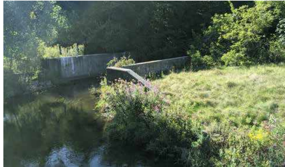
Existing Bridge abutment over Ore Creek
