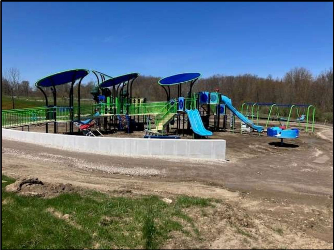
Picture: Progress at the Indian Springs Playground, from April 25th
