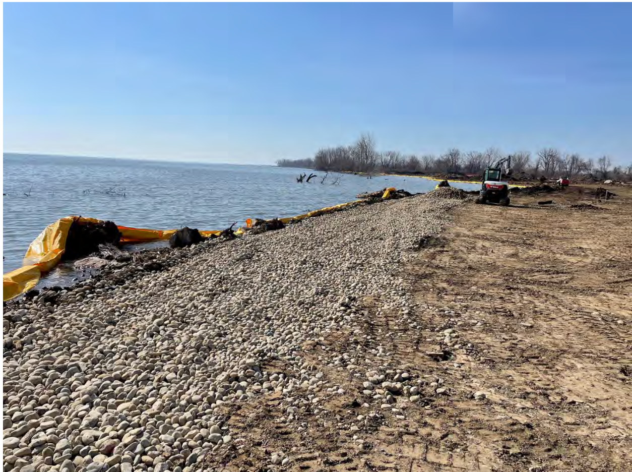
Figure 2: Shoreline restoration project at Lake Erie Metropark has largely been completed. This photo shows the new grade of the shoreline and the creation of a stone beach at the toe of the slope. Areas further upslope will be restored with a mix of wetland and wet-prairie vegetation.
