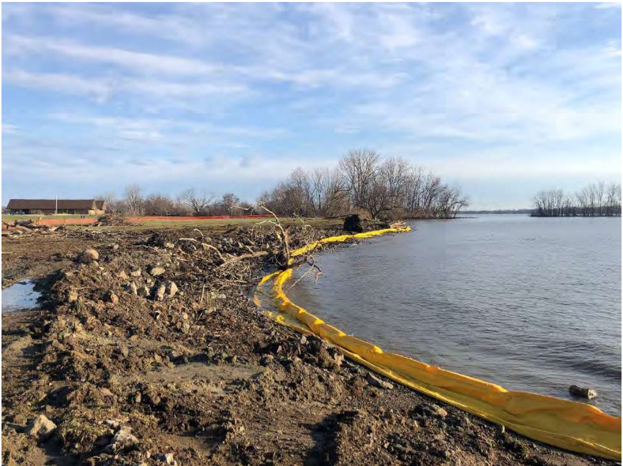
Figure 2: Shoreline restoration project at Lake Erie Metropark has begun. The shoreline has been graded to soften the slope, concrete rip rap has been removed, and woody debris has been incorporated.
