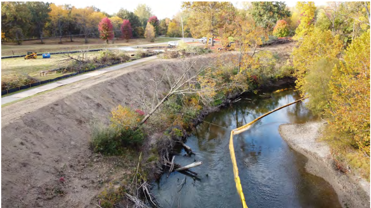
Figure 2: Bank stabilization and restoration at Willow Metropark in progress. Spring and Summer 2023 activities include planting of riparian buffer with native plants and trees..
