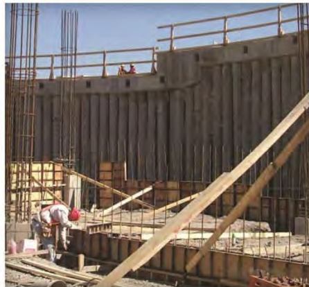
Earth Retention Wall Design and Construction
