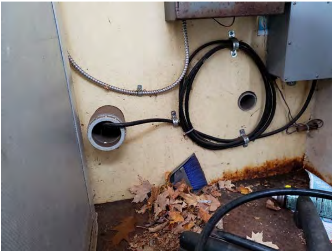
Lower Huron Fiber-Optic Installation
