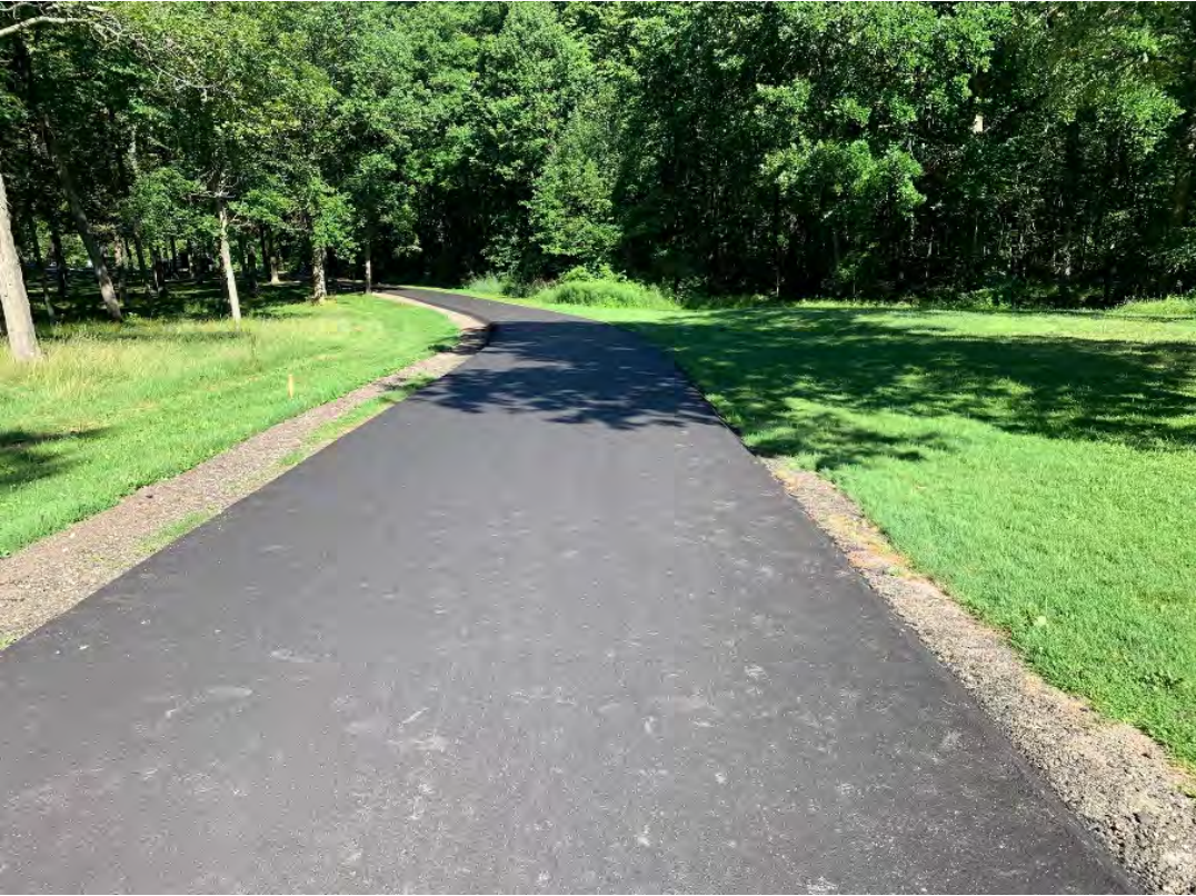
Hudson Mills Trail Reconstruction
