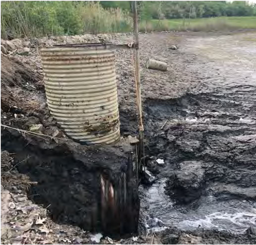
L-shaped control structure at the North end of the pond
